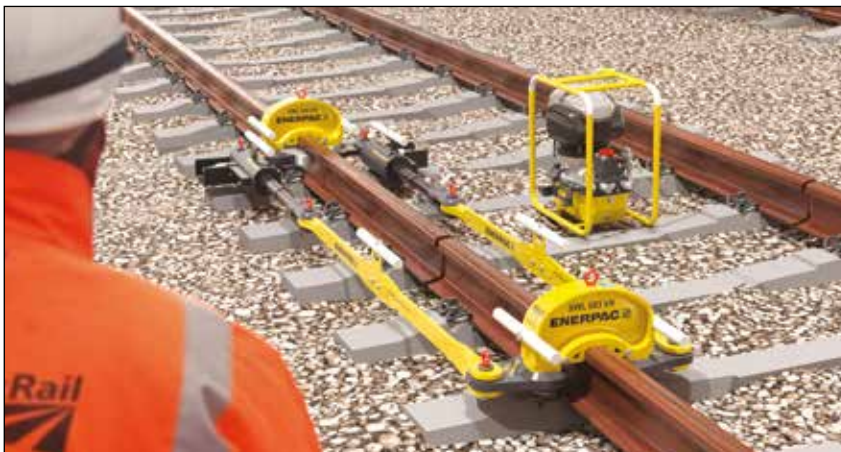
◀ Complete system with RP70A Hydraulic Rail Stressor and ZC3 cordless stressing pump.
