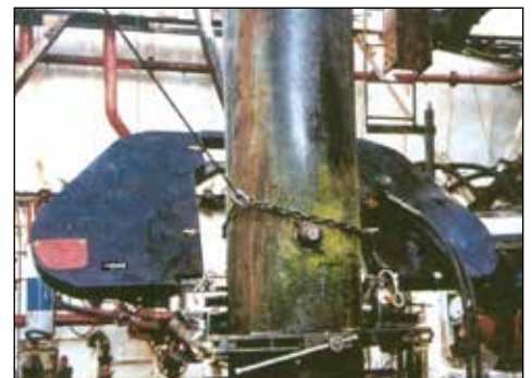
▼ Decommissioning job with band saw.
